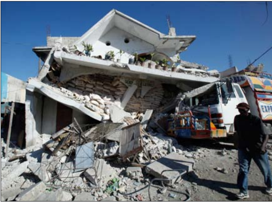
A Haitian man walks past a destroyed building in a suburb of Port-Au-Prince on Jan. 17, 2010. Decades of political corruption have led to shoddy construction of buildings that were unable to withstand the shocks of the earthquake.
