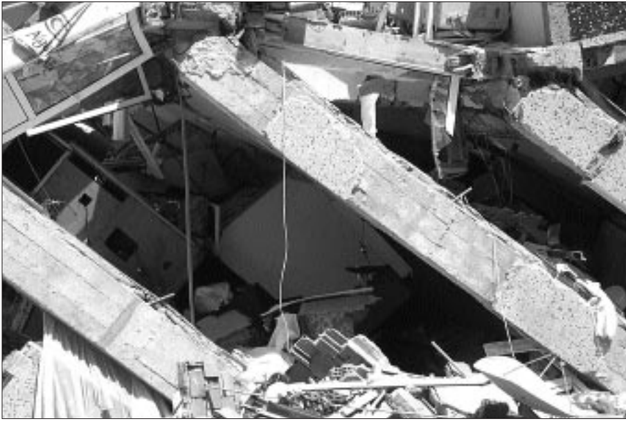
Devastating earthquakes topple concrete buildings like a house of cards
